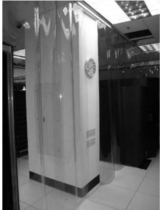
Figure 5: Working around obstructions
