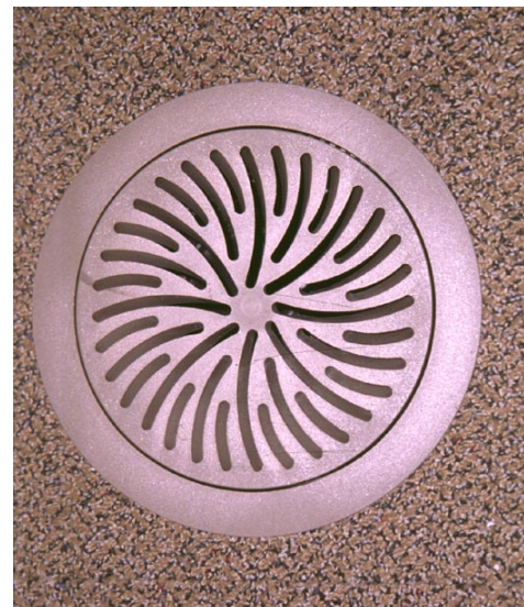
Figure 3. The Owens Corning headquarters building features an underfloor air plenum with Titus™ swirl-plate diffusers providing a flow rate between 0 and 90 cfm each.
