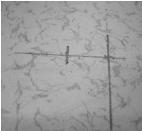
Figure 19: Mark 12" away from door jam
