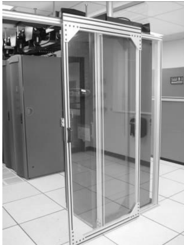
Figure 17: Adjusted sliding door assembly
