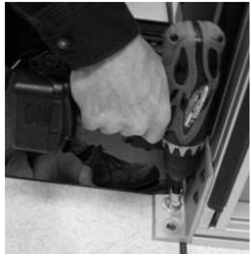
Figure 11: Drill the floor
