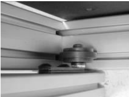
Figures 15 and 16: Door roller adjustments
