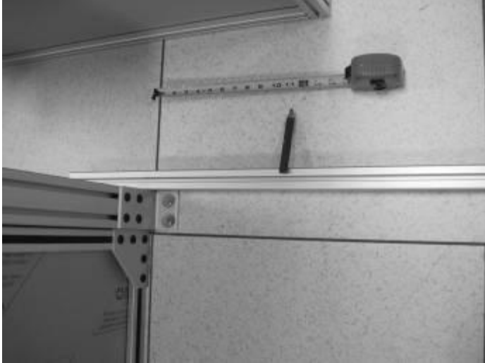
Figure 18: Floor guide installation
