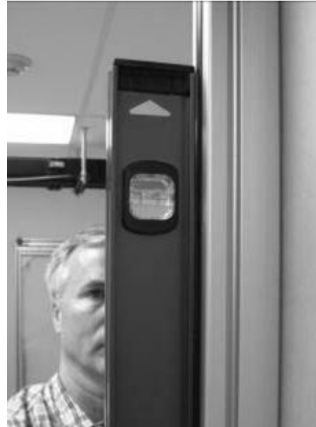
Figure 10: Plumb The doorframe
