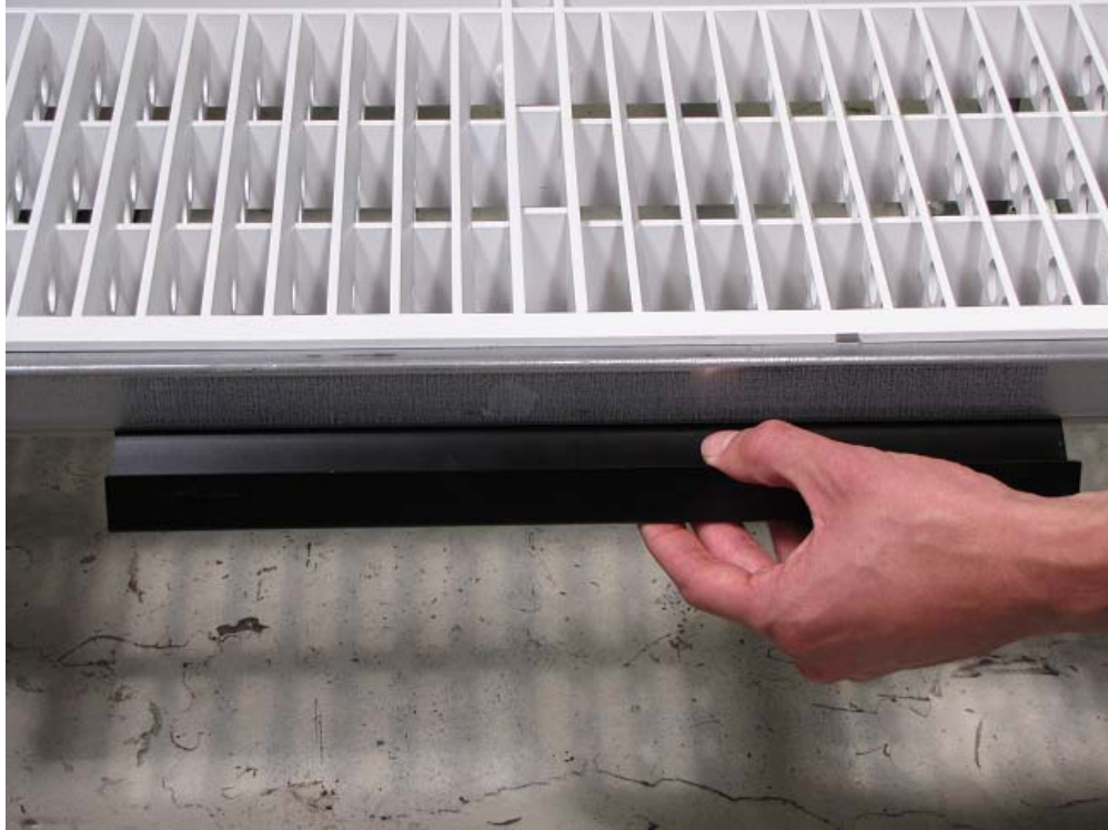
Figure 6 - Insert hanger into roll form opening and catch the top angle inside the stringer
