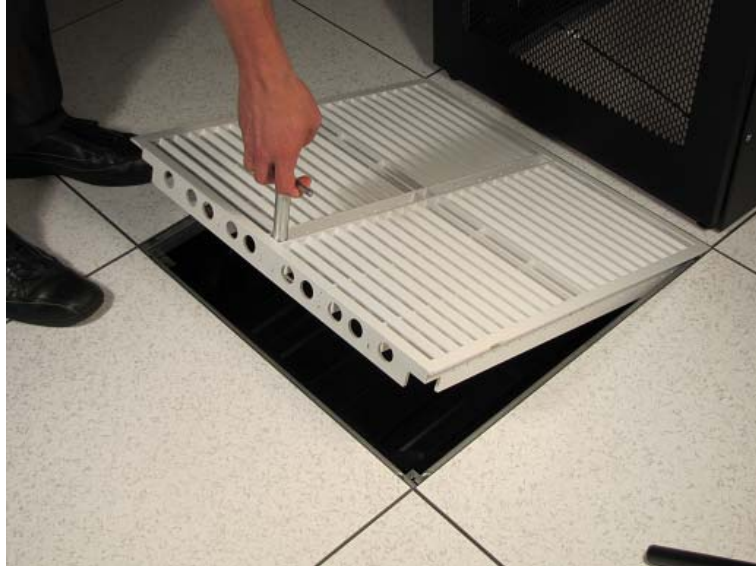
Figure 23 - Installation of DirectAire Panel
