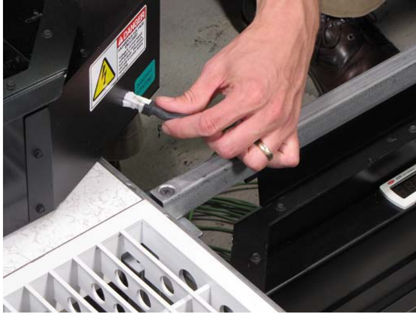
Figure 14 - Connecting next SmartAire from neighboring unit
