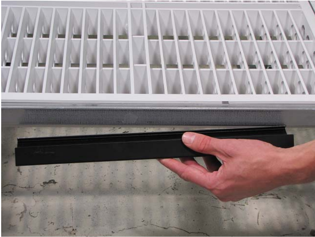
Figure 5 – Step 1, position hanger parallel to the floor with short angled edge aligned to opening in roll form stringer
