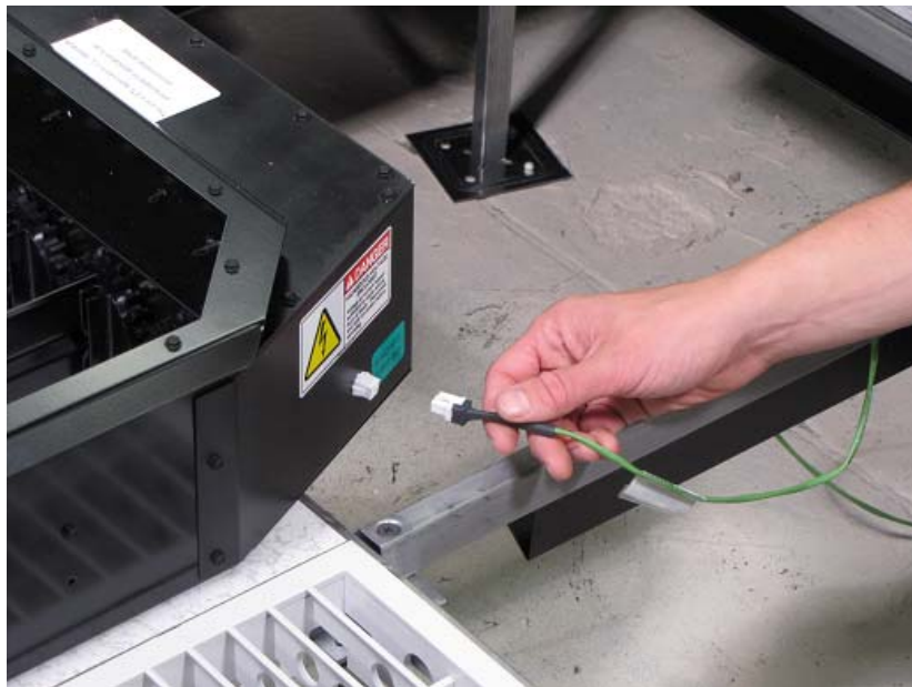
Figure 11 - Connecting LV power to SmartAire Unit
