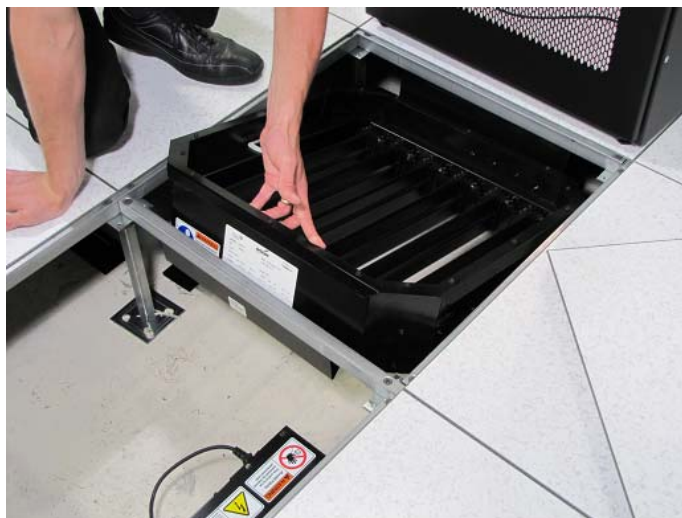
Figure 15 - Installing SmartAire unit into Floor
