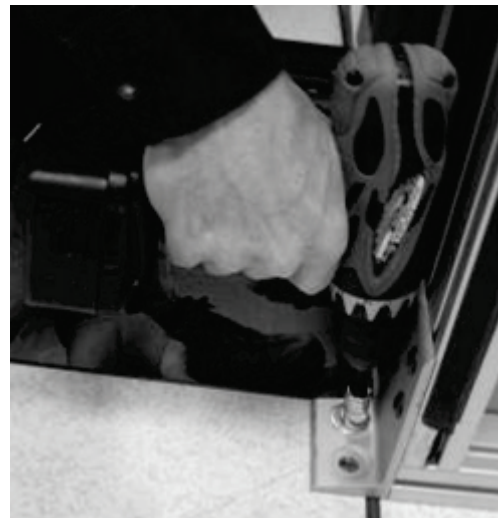
Figure 4: Drill the floor
