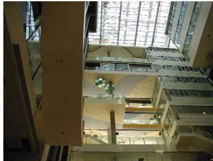
The Genzyme Corporation's recently completed office in Cambridge is a world-class example of green building construction, including advanced daylighting and thermal technologies. In addition to a photovoltaic installation funded by MTC, one of the most prominent features is a combined heliostat and reflective panel system designed to channel daylight deep into the 8-story building.
