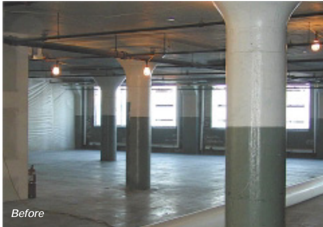
Construction involved integrating original architectural features, such as columns, and modern technology requirements into an aesthetically pleasing, energy-efficient workspace
